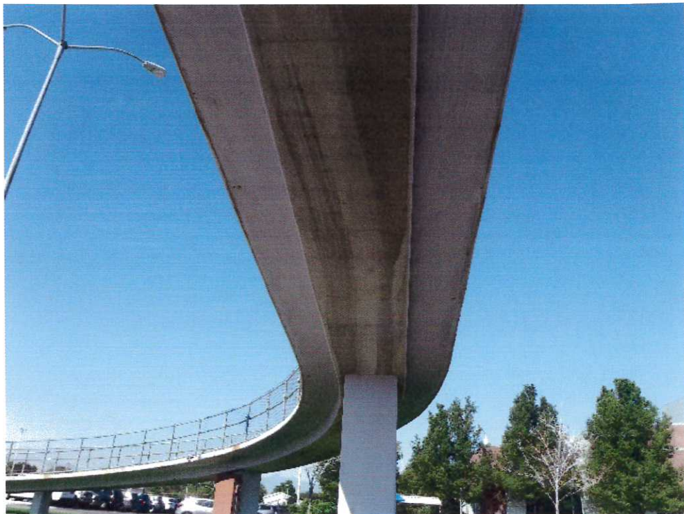
Figure 10 - Underside of Concrete Girder and Deck
