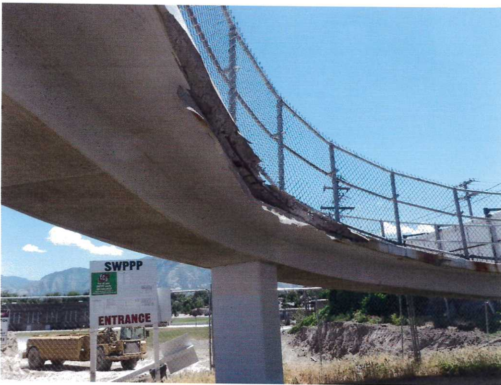
Figure 8 - Spalling and Exposed Reinforcing of Deck Overhangs
