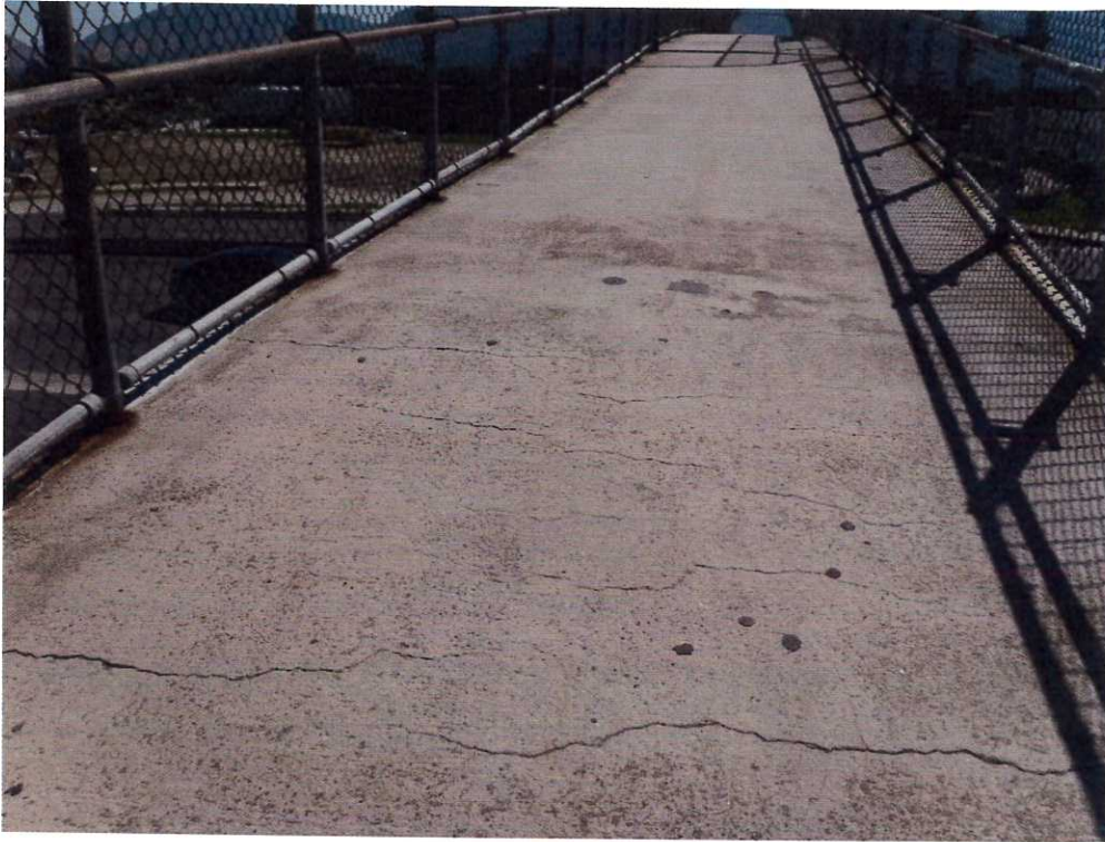
Figure 7 - Deck Surface - Cracking, Abrasions, Fence Corrosion
