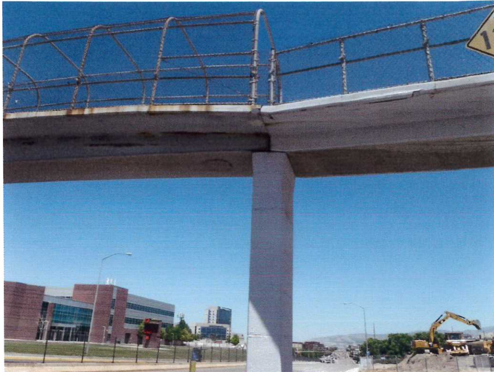
Figure 9- Steel Girder (left), Concrete Girder (right), Pier #6
