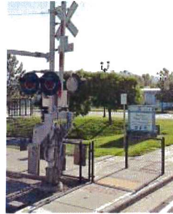
Current crossing arm configuration at the TRAX Station and Winchester Street. Note the conflict of the ADA truncated plate.
