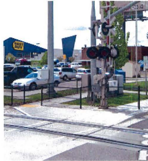
Figure 4.15 Example of improved crossing arm configuration at Central Pointe Station and 2100 South. The sidewalk is rerouted to ensure no conflict between pedestrian route and crossing arm.
