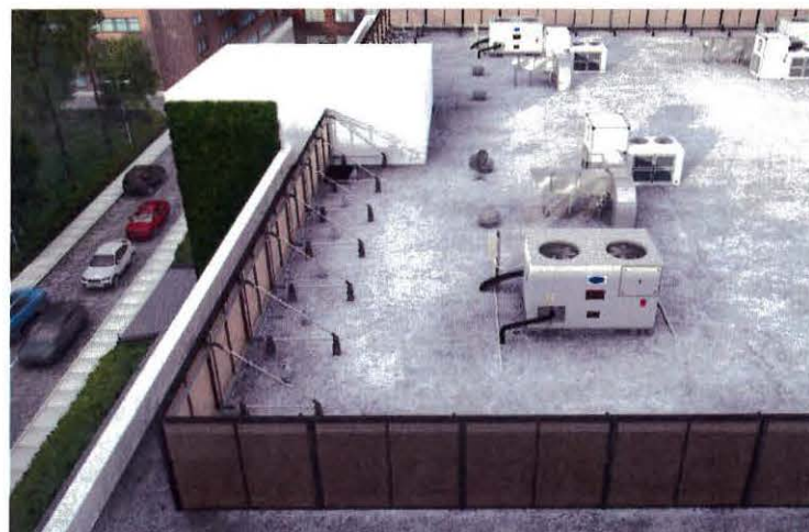
Figure 5.16 Buildings that require utilities or mechanical equipment to be positioned on the roof, should be screened from public view using materials complementary to the building facade and the surrounding neighborhood.
