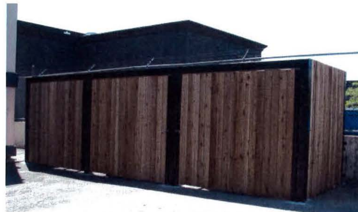
Figure 5.15 Waste containers and dumpsters should be shielded from view using permanent materials. This screening should decrease the visibility and visual impacts of these types of areas.
