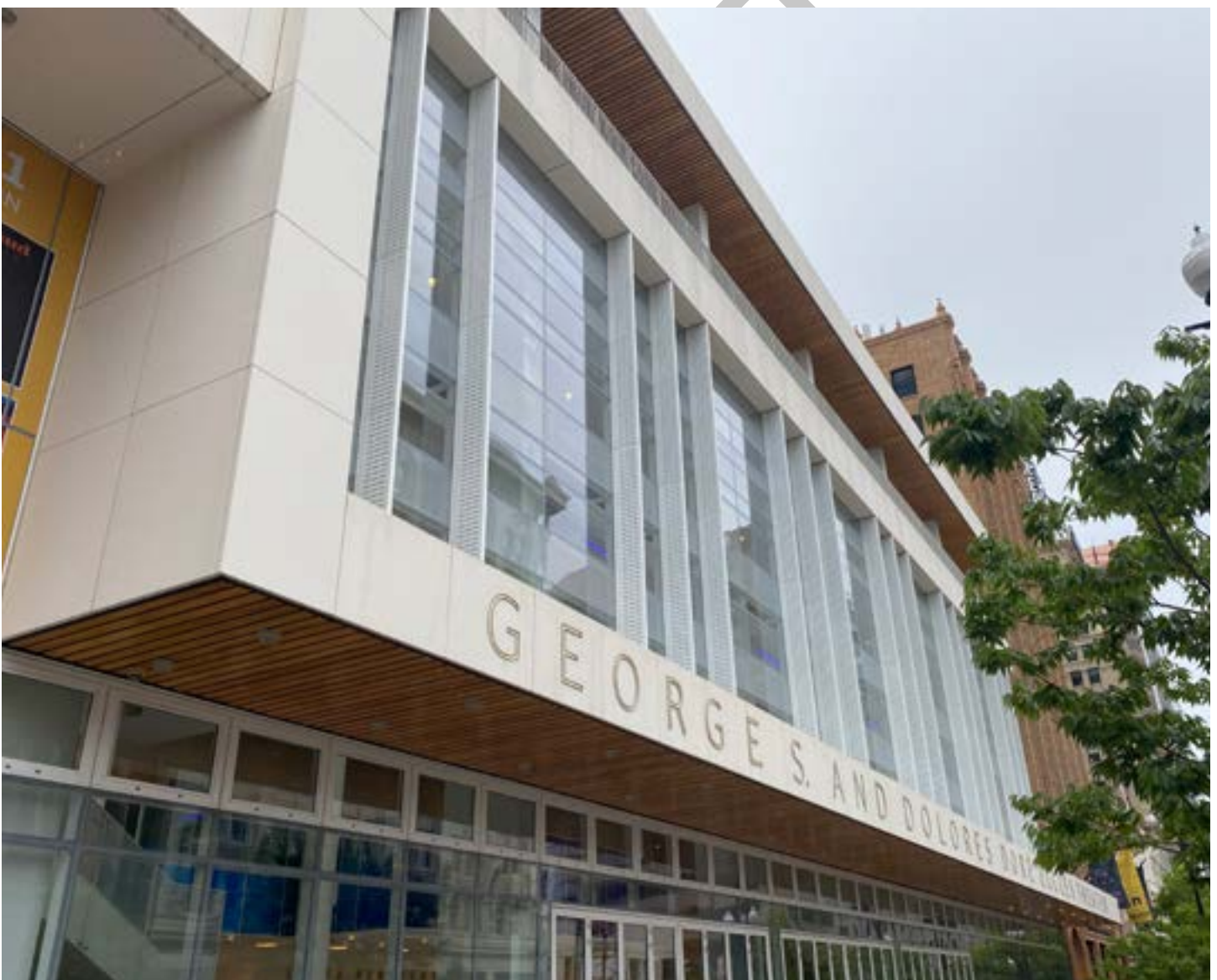
Contemporary building with depth and texture, the fins on the windows are used as a passive solar device to help shade the interior of the building.
