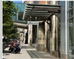
Incorporating shade structures along pedestrian paths reduce the amount of heat put off by a building and reduces energy use.
