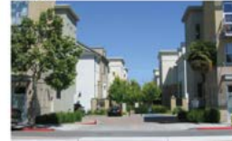
In this project, commercial and residential parking is accessed using one driveway, which minimizes the number of entrances and exits to parking areas and reduces conflict with pedestrians. (Guideline G-1)
