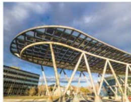
Shade structure outside of the Salt Lake City Public Safety building also serves as a solar power generator.
