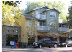
The taller stories of this project are located in the middle of the project which minimizes the impact of the project on adjacent neighboring property. (Guideline A-2)
