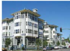
This project provides architectural interest and enhances the visual appearance of the street. (Guideline A-1)
