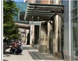
Incorporating shade structures along pedestrian paths reduce the amount of heat put off by a building and reduce energy use.
