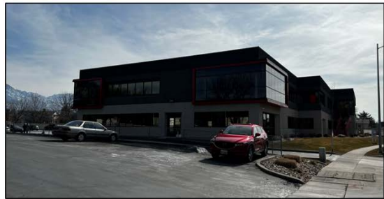
Photographs of several office buildings and complexes in the G-O Zone.
