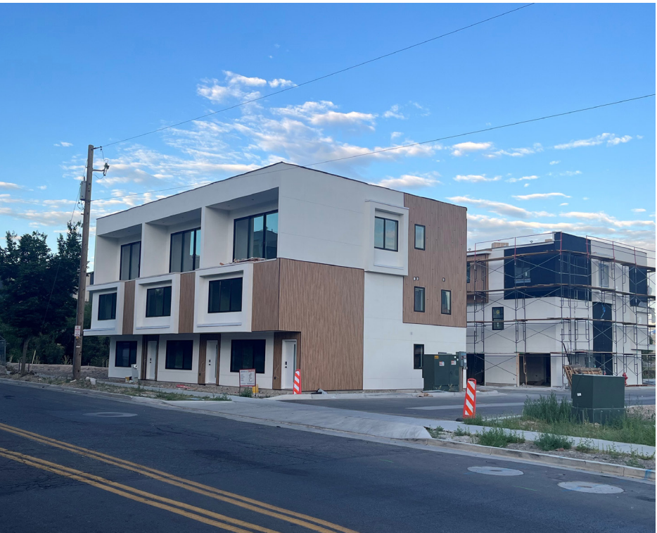
FIGURE 2.5: HOUSING UNDER CONSTRUCTION ALONG MAIN STREET
