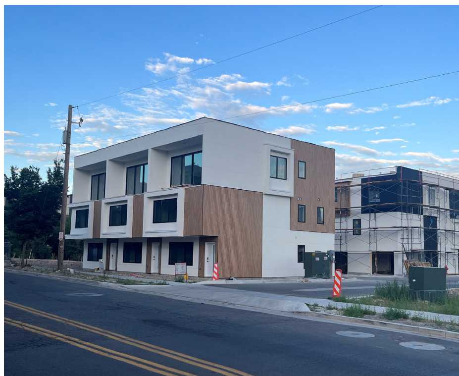
FIGURE 2.5: HOUSING UNDER CONSTRUCTION ALONG MAIN STREET
