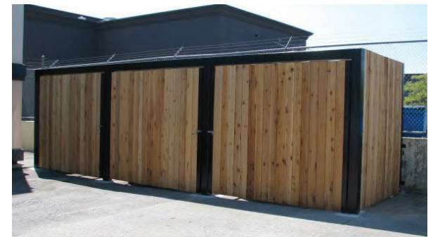
Figure 5.15 Waste containers and dumpsters should be shielded from view using permanent materials. This screening should decrease the visibility and visual impacts of these types of areas.
