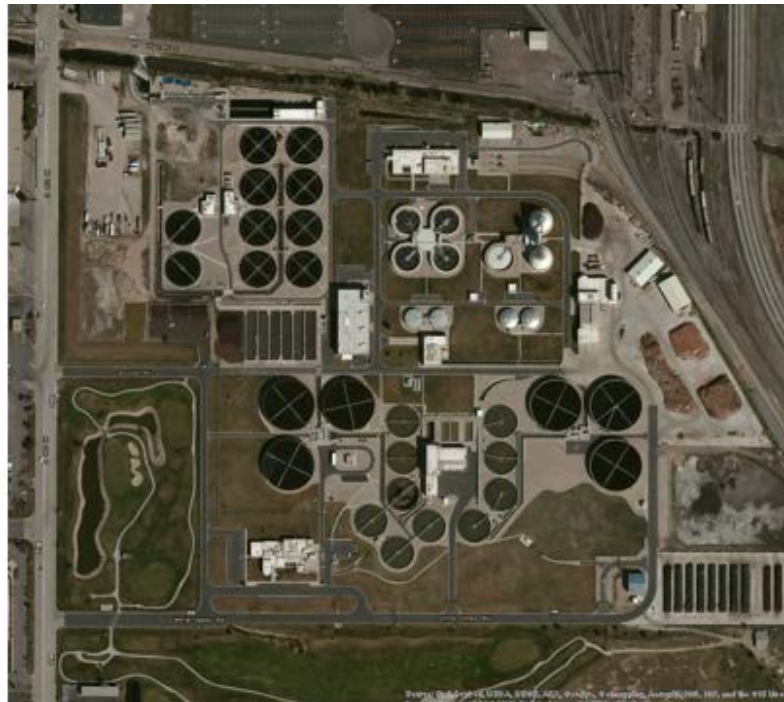
Central Valley Water Reclamation Facility
