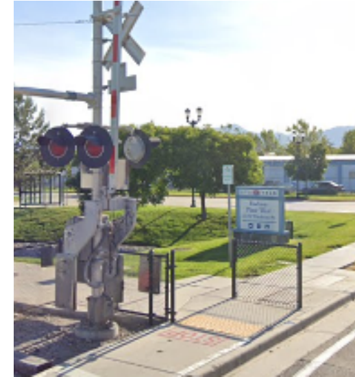
Figure 4.16 Current crossing arm configuration at the TRAX Station and Winchester Street. Note the conflict of the ADA truncated plate.
